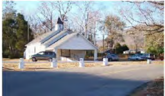
View of the building from the road approaching the church
